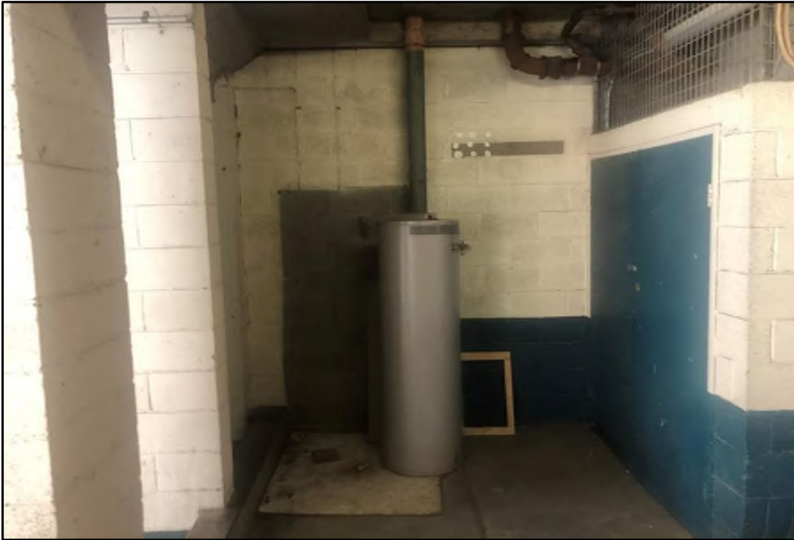
Photo 9: Hot water system in basement of No 52-56
